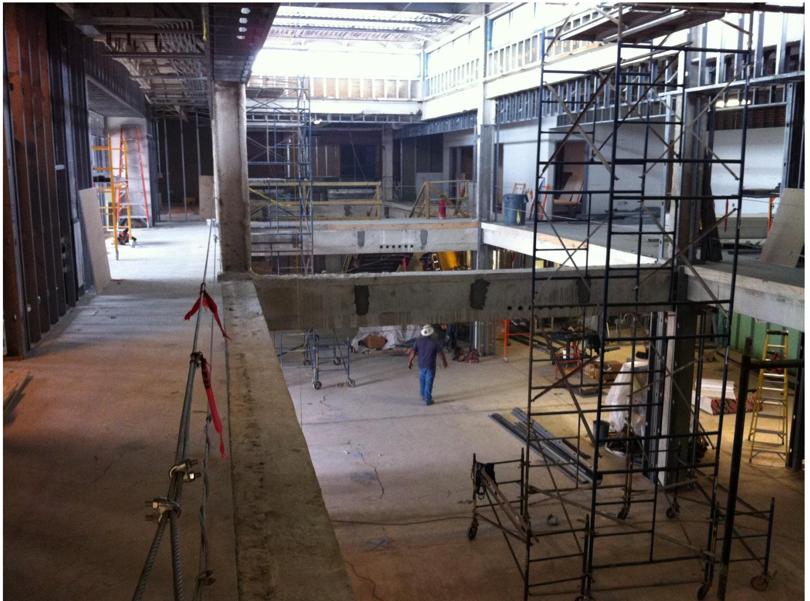
“The Ring” under construction – looking north
