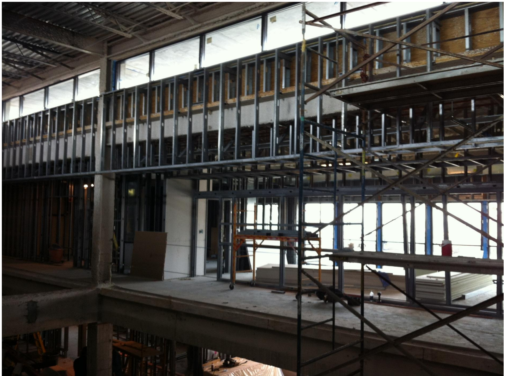
“The Ring” under construction – west side
