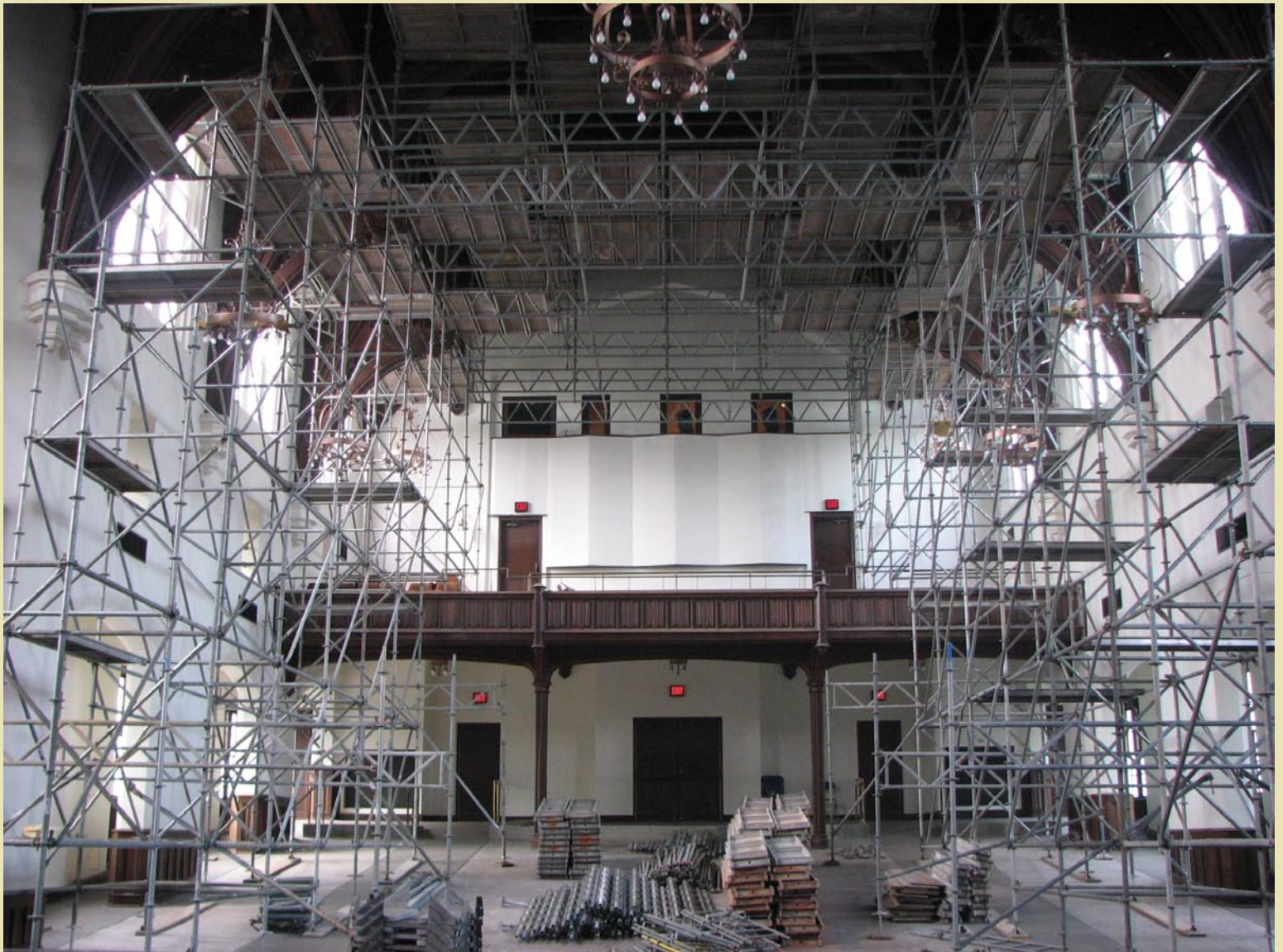
The University Auditorium under renovation in summer 2007.
